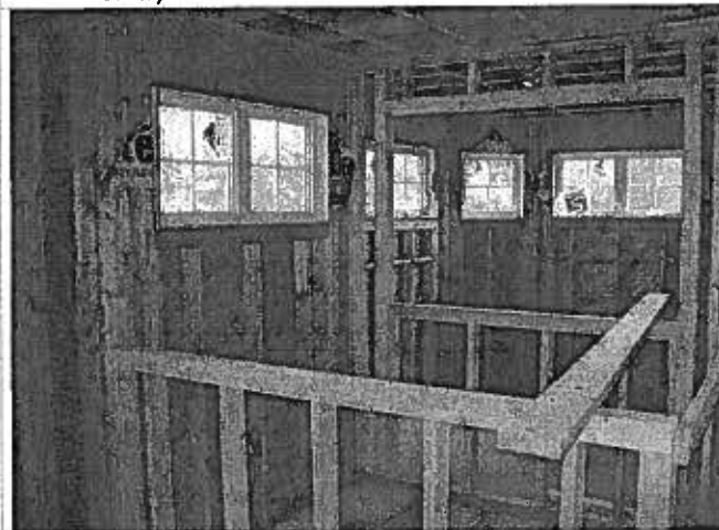
33. Unit 59 under construction (library)
