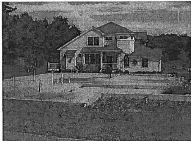
9. Unit pad installed
