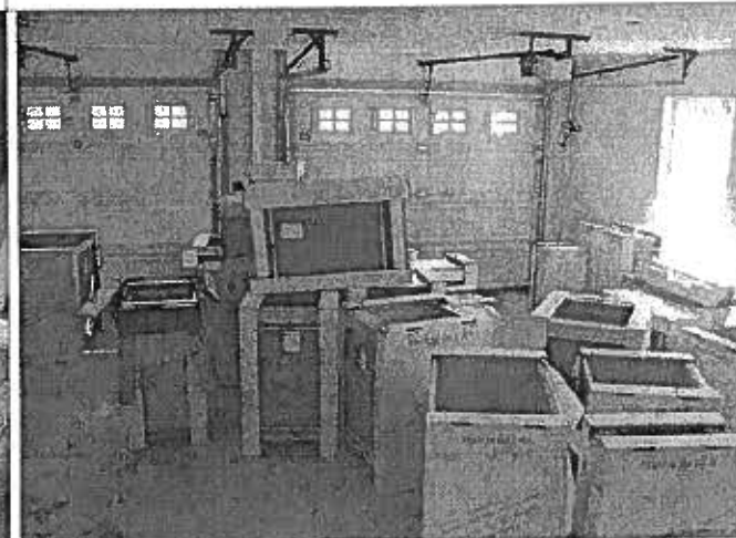
36. Unit 58 under construction (kitchen cabinetry staging)
